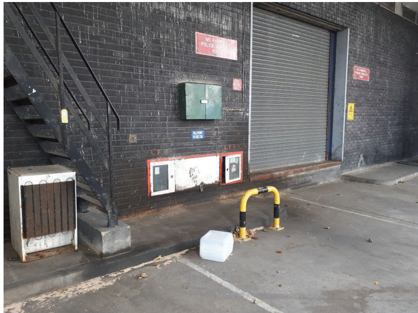
Photo 6. Tank fill point in the east of the site, likely associated with oil fuel heaters formerly located in the eastern extent of the basement.
