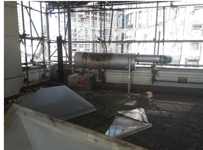
Photo 8. A 'silencer' and associated generator on the flat roof of the elongated low-rise structure connecting the eastern and western towers.
